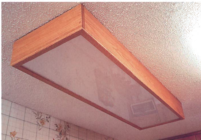
Don't overlook lighting requirements when converting your closet into a work center. Fluorescent fixtures are ideal and the looks can be improved upon with a few boards and a sheet of 1/8"-thick Plexiglas. Build a box using 1x6 material, add moulding to the bottom edge that's wide enough to create a 1/4"-wide inside lip, and slip in the Plexiglas panel.
